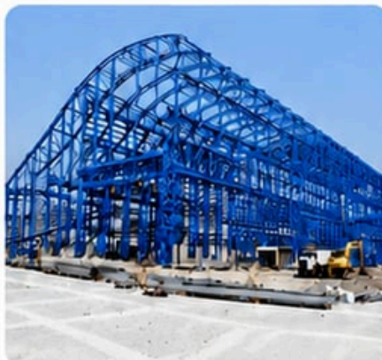
BUILT UP CURVED RAFTER
